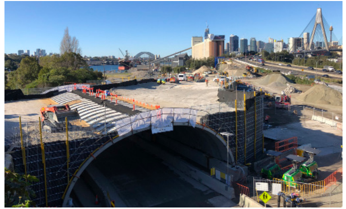
Sydney, Australia: TechSpan® precast concrete arch used for the M4 WestConnex tunnel.
