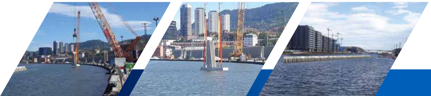
TechWall™ installation underwater
