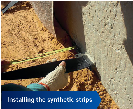
Installing the reinforcements
