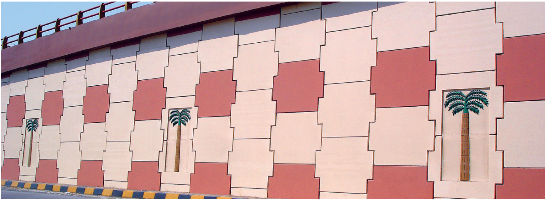
Navghar Flyover, Mumbai International Airport Mumbai, India ▶
