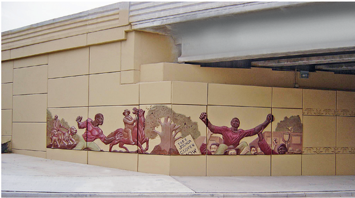
Marquette Interchange Milwaukee, Wisconsin, USA ▶
