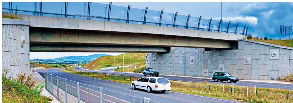
Oak Flats Interchange, South Coast
