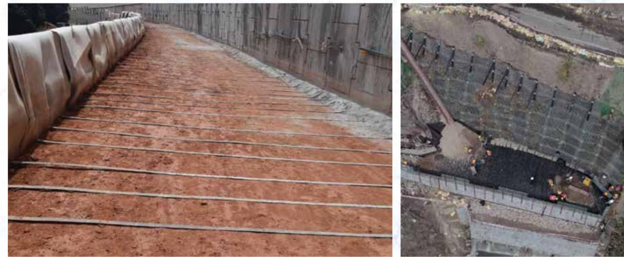
**Shored MSE®** technique allows building of earth retention structures connecting existing profiles stabilized by soil nails and/or anchors. It is a useful technique for construction of benches and for road widening projects with limited available space, and activates the best optimisation between cut and fill requirements.
