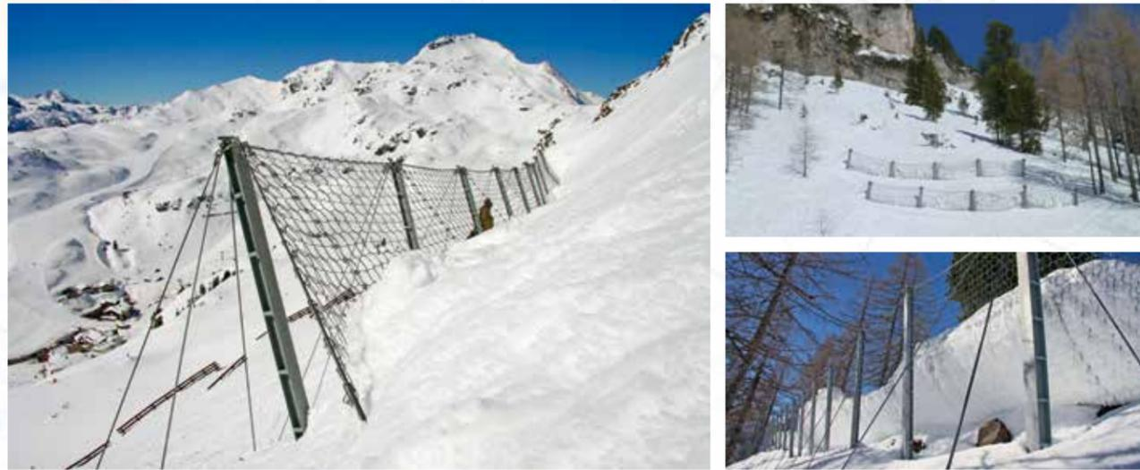
**Avalanche Barrier** systems are designed on a site-to-site basis to protect infrastructure, utilities, buildings, reforestation, and lives from avalanches. Snow nets, snow rakes and steel snow bridges are installed in the initiation zones to prevent avalanches from forming. Static defense structures, snow catchment fences/barriers are used which effectively reduces the run-out length of an avalanche.
