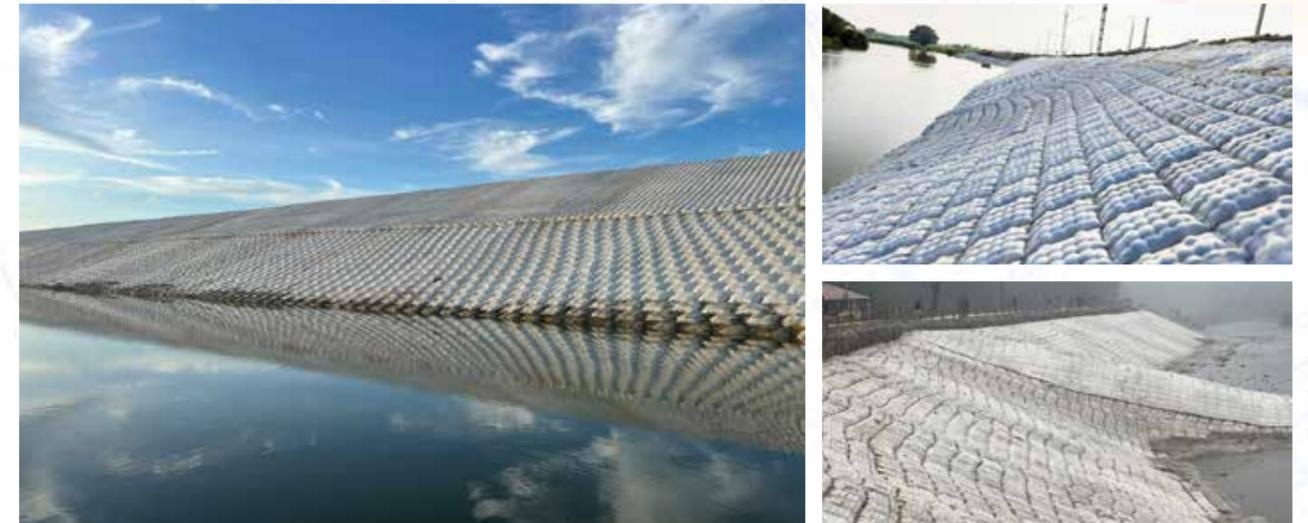
**TechRevetment®** is a pre-engineered factory costumed grouted mattress system used for permanent erosion protection works. This technology is used to protect embankments, protect bridge abutments against scour, for bed protection of major rivers and waterways, and for shoreline protection. This system can be installed at rapid speed and under water without the need for dewatering.
