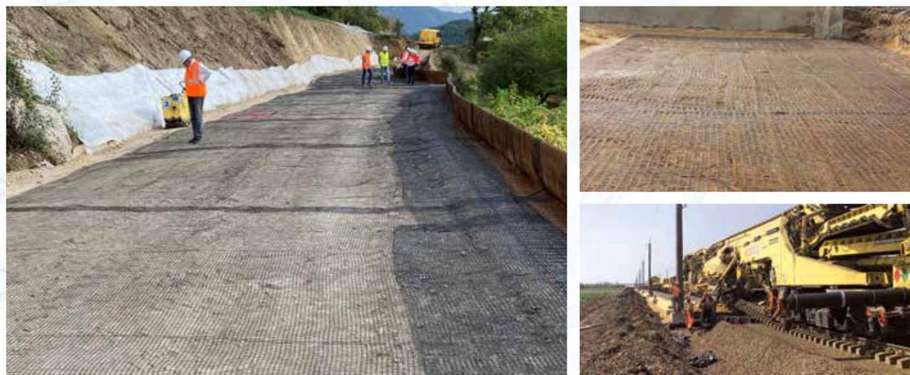
**ArmaGrid™** is a uniaxial or biaxial geogrid made from either polyester or polypropylene or HDPE. It is used as soil reinforcement in various applications such as foundation improvement, trackbed stabilization, basal reinforcement etc. The Reinforced Earth Company uses in-house design capacity to select the type and strength of material based on the actual site condition.
