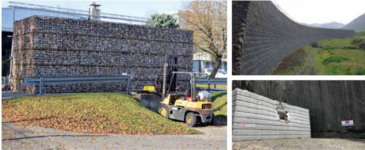
**TerraBund®** is a Terre Armée protection bund. It is a gravity structure built using soil reinforcement and flexible or semi-rigid facing systems. It is a passive protection system used typically as a geo-hazard solution against rockfalls, avalanches, debris flow and mud slides. **TerraBund®** can withstand more than 8000kj of impact energy in the event of landslide or rockfall.
