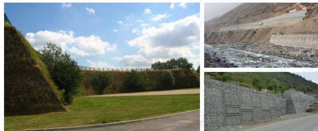
Reinforced soil slopes (RSS) are an extension of the Reinforced Earth® technique. These structures are designed and built to retain with a face inclination of between 45° and 70°. ArmaGreen is the name of our vegetated facing solution, while ArmaStone is the name when we use a mineral facing.
