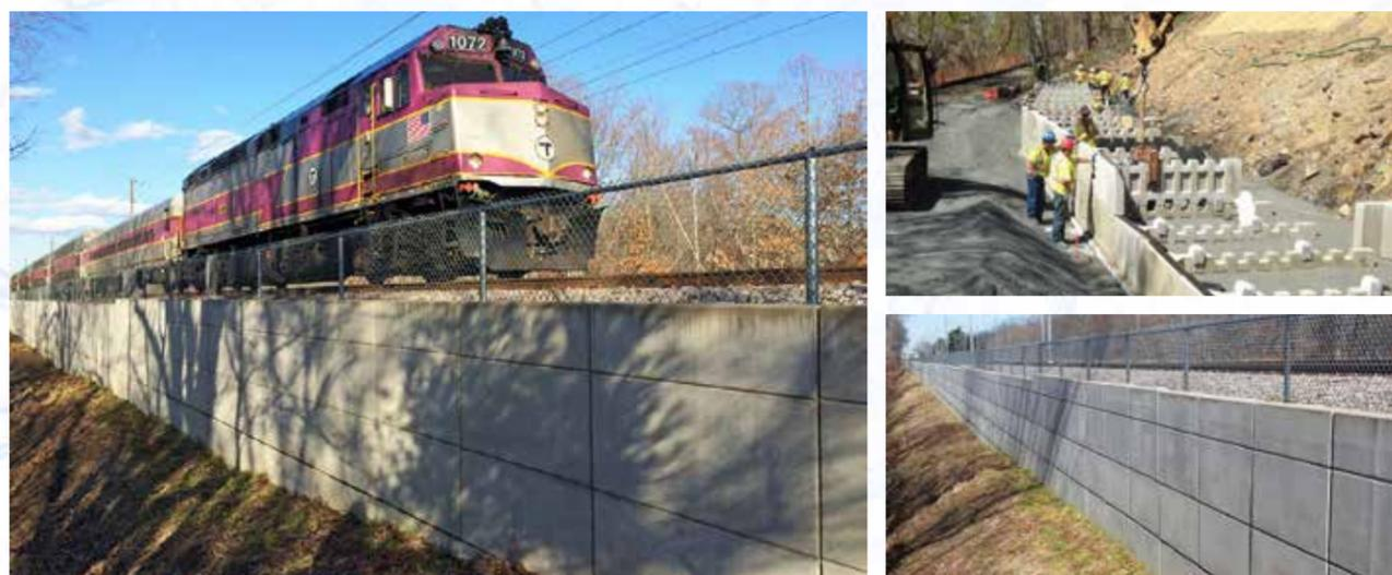
The **T-Wall®** system is a precast modular gravity type reinforced concrete retaining wall system. It is most suited for railway load supporting structures and construction of submerged retaining structures. The **T-Wall®** system decreases in stem length course by course – reducing materials, excavation and backfill as compared to other wall systems.
