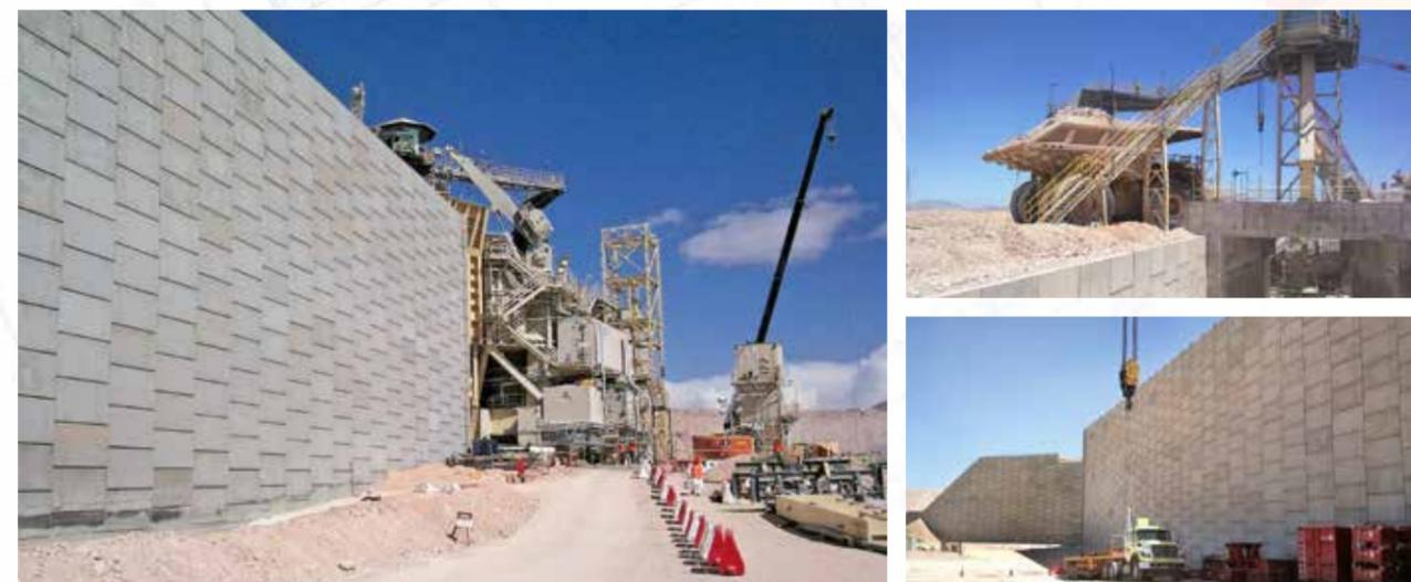
**Composite Earth®** technology adopts primary and secondary soil reinforcement systems for the design of Reinforced Earth® retaining walls. It aims to control the lateral deformation of the facing during construction and operation, including during seismic events. This is an effective way to design and construct tall and critical structures.
