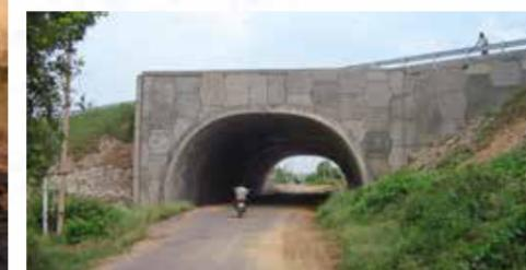
**TechSpan®** is a one of the most reliable, cost effective precast concrete arch systems available for cut 'n' cover structures. It is widely used in the construction of bridges, underpasses, conveyance and reclaim tunnels, portals, ammunition storage bunkers and rockfall sheds and shelters. Typically, 15-20 linear meters of **TechSpan®** can be installed in one work shift.
