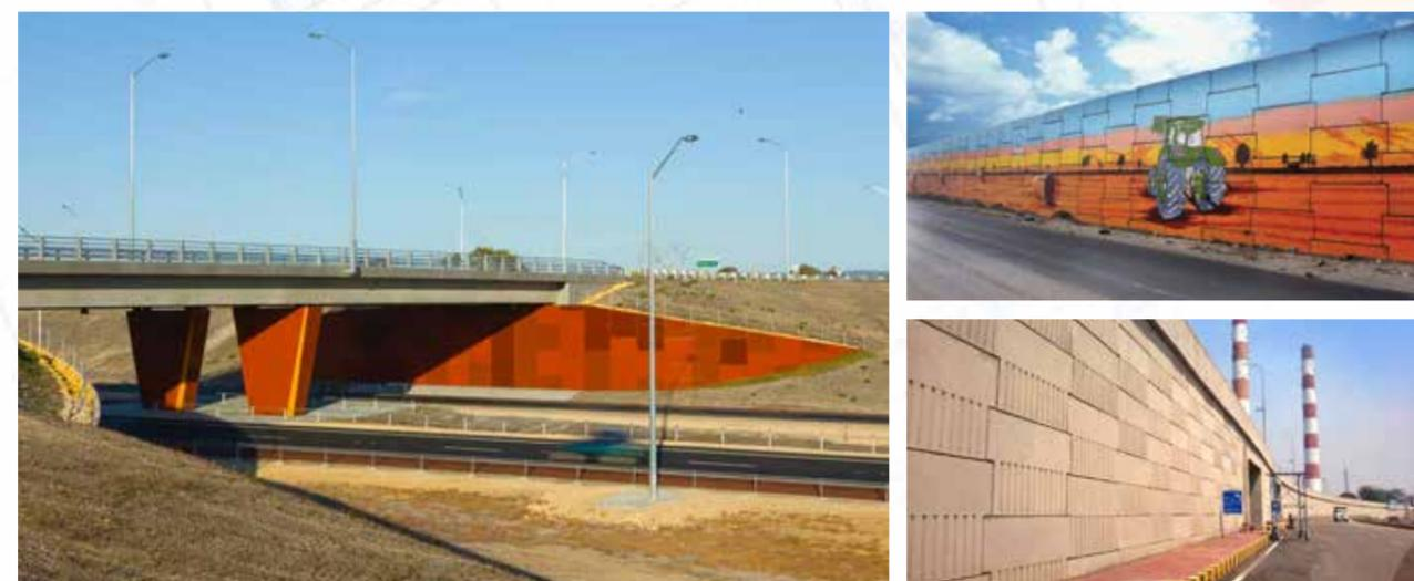
**Reinforced Earth®** structures combine engineered backfill with steel or synthetic tensile reinforcement and a modular concrete facing system. This ideal combination creates a durable and resilient earth retention structure. With **Reinforced Earth®** structures we can create several attractive architectural finishes.
