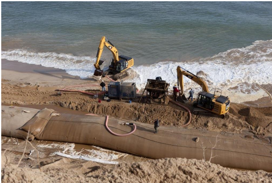
Left and above: Filling the TITANTube® geotextile tubes with the dredged sand
