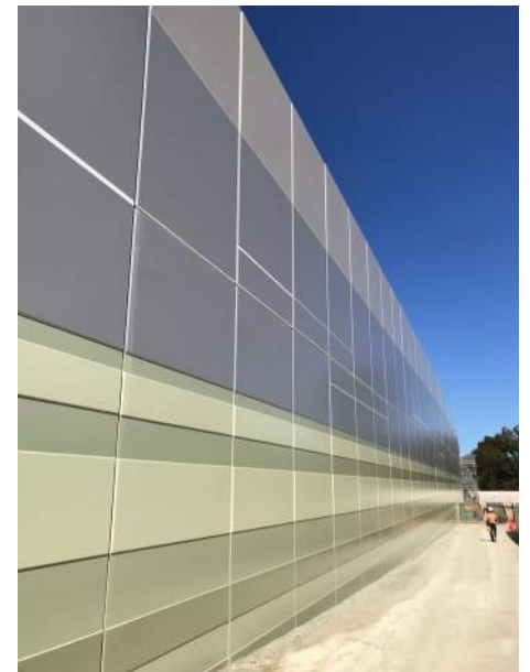
Reinforced Earth TerraTilt walls Stacked one on top of the other - with screen wall extension
