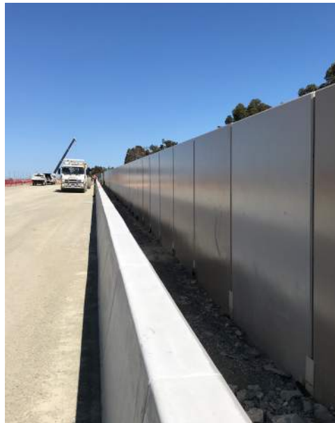
Screen wall extension - viewed from behind the walls
