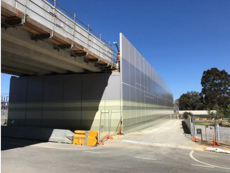
Reinforced Earth TerraTilt Abutment
