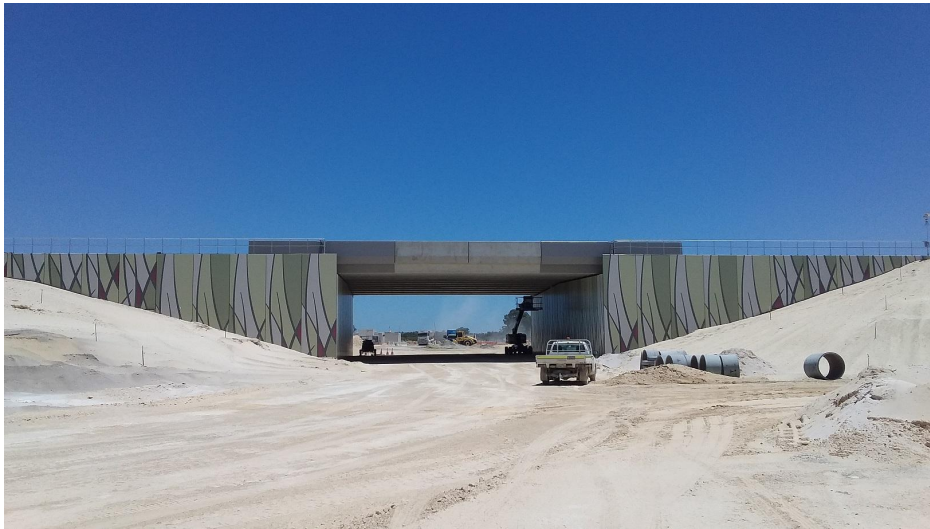
Bridge 1793 - TerraTilt Abutments and Precast Parapet Barriers
