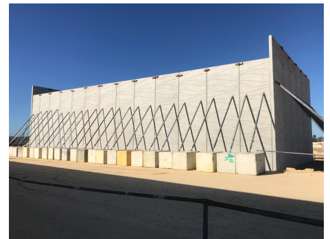
Bridge 1802 - TerraTilt panels propped and ready for backfill
