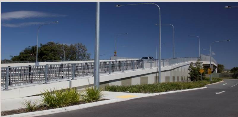
Left: The completed structure of Francis Rd Rail Overpass
