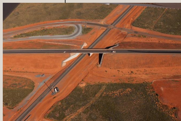
Above: Aerial View of the road bridge over the BHP Billiton Railway Line
