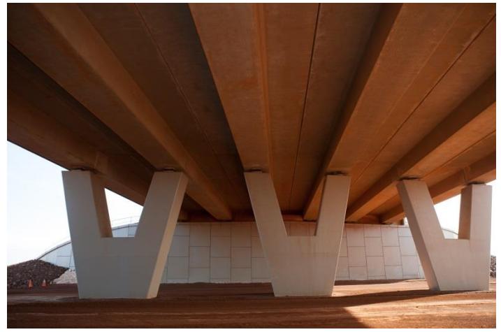
Above: Reinforced Earth® Bridge Abutment, part of the Interchange Bridge
