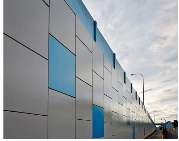
Above: Reinforced Earth® TerraPlus® Retaining Walls with Painted Finish. Photographs courtesy of John Holland
