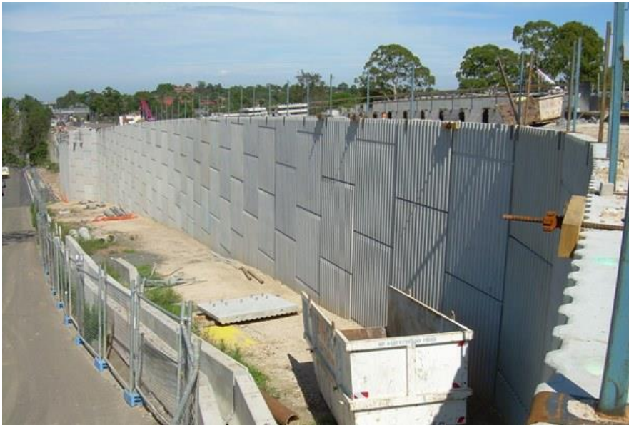
Left: A completed section of the TerraPlus® panel wall with a vertical rib finish Above: A completed section of the TerraTee® wall built on difficult terrain.
