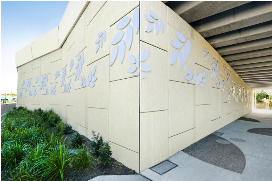
Left: TerraPlus® Reinforced Earth® walls at the Ipswich Motorway Upgrade – Dinmore to Goodna. This is part of the 'leaf' pattern. Above: Construction of the Reinforced Earth® walls with the wave pattern, Dinmore, NSW.
