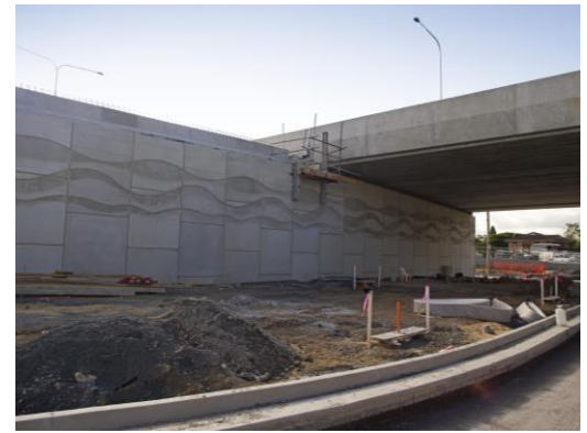
Left: TerraPlus® Reinforced Earth® walls at the Ipswich Motorway Upgrade – Dinmore to Goodna. This is part of the 'leaf' pattern. Above: Construction of the Reinforced Earth® walls with the wave pattern, Dinmore, NSW.
