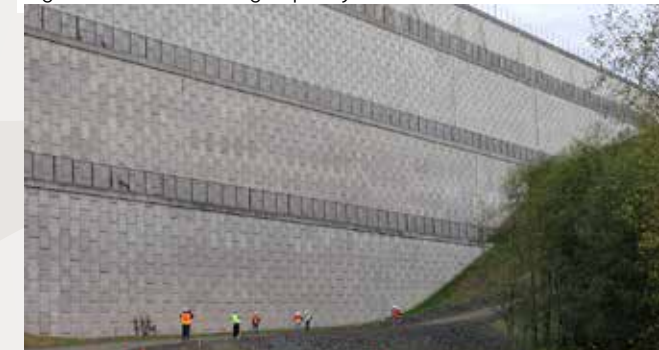
45 meter high tiered wall - SeaTac airport - USA
