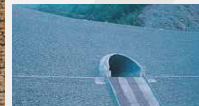
Inclined wire mesh facing
